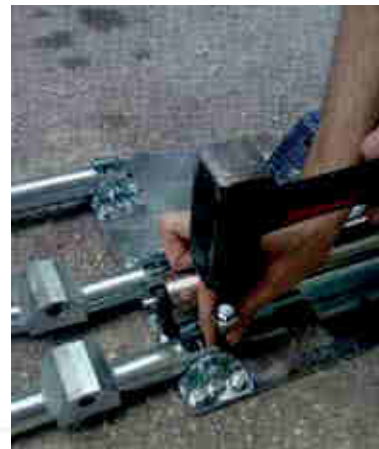
Figure 10 - Anchor placement
