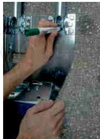
Figure 8 - Marking drilling spots
